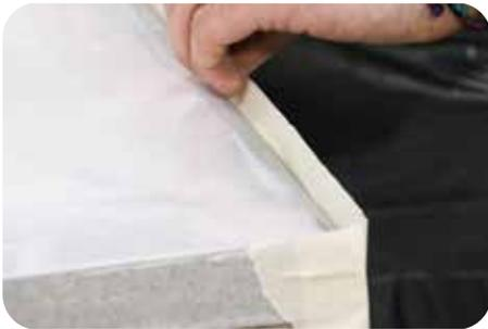
Replace the masking tape you removed from the back edge and underneath the front edge, repeating the same positioning and technique as before.
