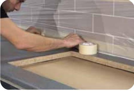
You will mask off once for the primer coat and then remove and replace this masking tape for the main pour. In both cases, you will be removing the masking tape before the resin cures.
