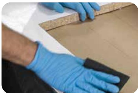
Once the resin is hard and dry, key the surface thoroughly with 120 grit abrasive paper by hand. We don't recommend using a power sander for this stage. Make sure you don't miss anywhere, including into the back corners and all the way over the rolled front edge.
