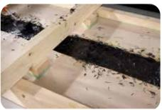
Next use a combination of brush and roller to mix the tow into the resin.
