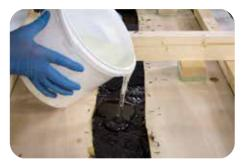
Pour the clear resin on top of the previous layer, filling up to approximately 5mm below the top of the planks. Saving a small amount of the mixed resin in the bucket for top up's.
