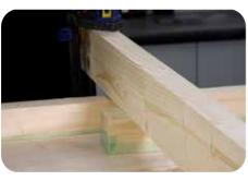
When applying the tape to the batten leave an overhang, fold it back on itself to create a crease and use this to stick it to the base sheet.
