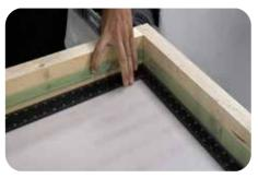
To create the barriers around the perimeter of the slabs of sycamore, use some wooden battens and resin release tape.
